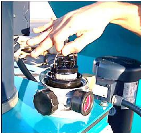
Step 2 – Pull out filter and install new
